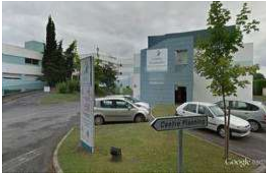
Centre hospitalier (source : Google earth)
