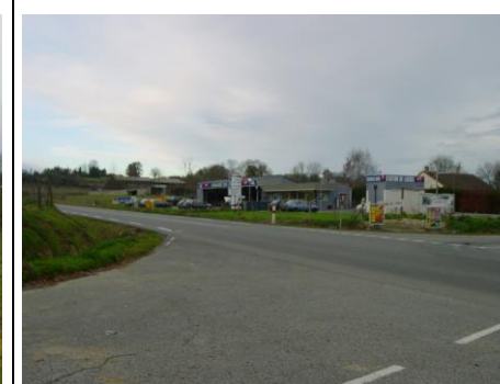
Station de lavage
