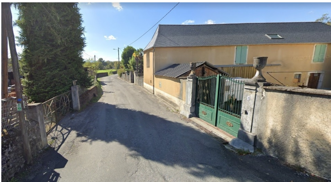
Front urbain existant rue du Gave
